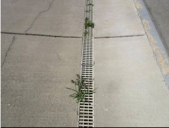
Drain Full of Debris
