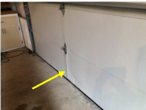
Dented/Damaged Overhead Garage Door
