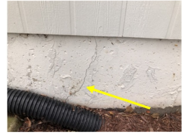
Common Foundation Crack(s)
