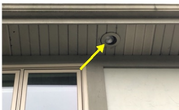
Loose Soffit Light
