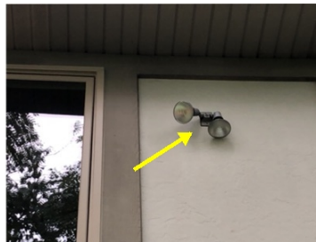
Loose/Damaged Flood Light (Back)
