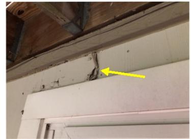
Loose/Damaged Siding
