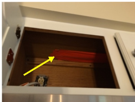
Abandoned Exterior Exhaust
