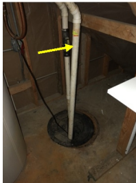
Loose Plumbing Vent Pipe
