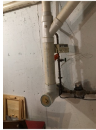
General View of Drain Clean Out
