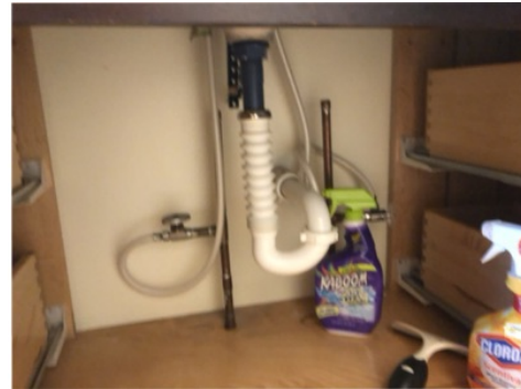
Ribbed Drain Pipe (Left Sink)
