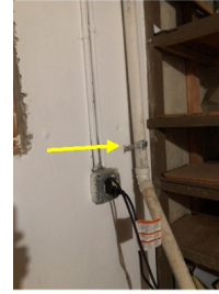
Loose Sump Pump Piping
