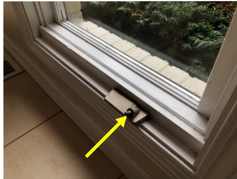
Missing Window Cranks
