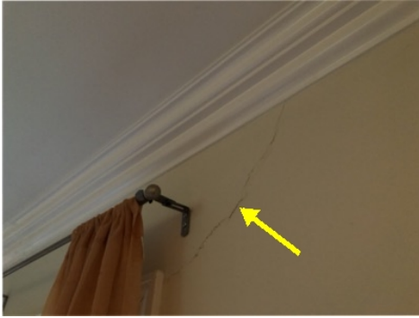
Typical Settlement Cracking
