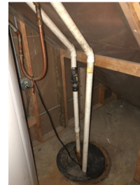
General View of Ejector Pump
