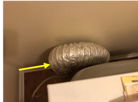
Improper Dryer Vent Material
