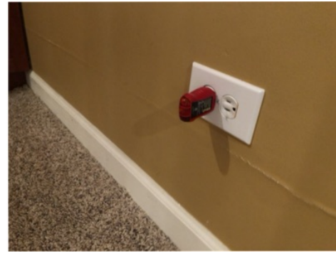
Dead Outlet (Bottom of Basement Steps)
