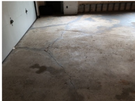
Typical Cracking
