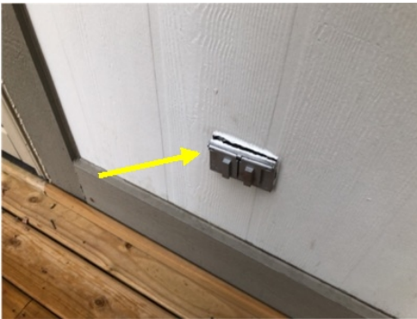
Loose/Damaged GFCI
