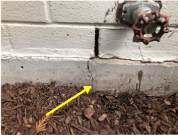
Common Foundation Crack(s)
