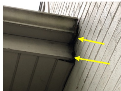
Deteriorated Soffits and/or Facia
