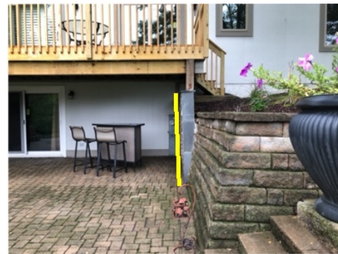
Leaning Retaining Wall
