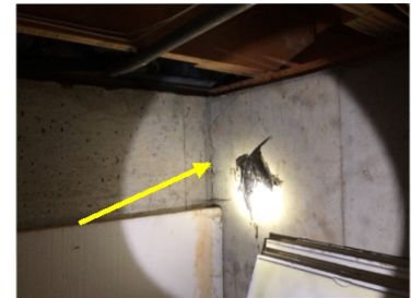
Possible Structural Movement
