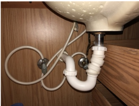
Leaking/Flex Drain (Right)
