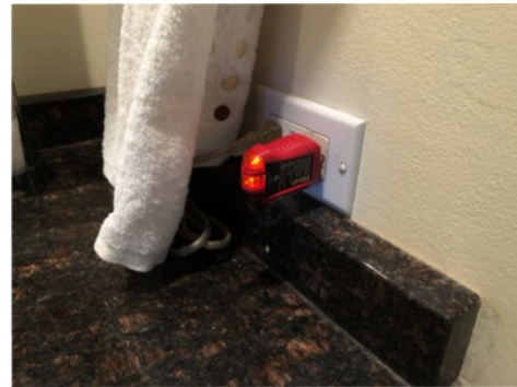
Failed GFCI (Master Bath)
