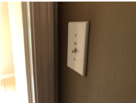
Loose/Worn Switch (Family Room)
