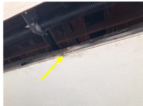
Damaged Weather Guard
