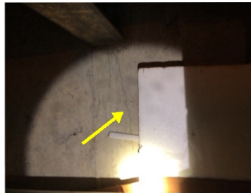
Typical Cracking
