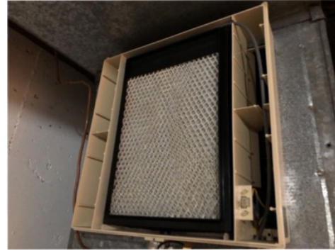
General View of the Humidifier Pad
