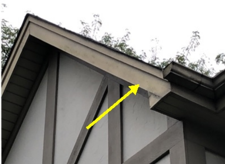
Paint Failure/Fading
