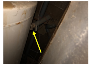
Missing TPR Valve Extension
