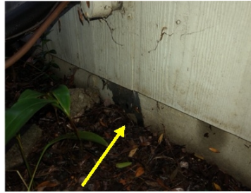
Common Foundation Crack(s)
